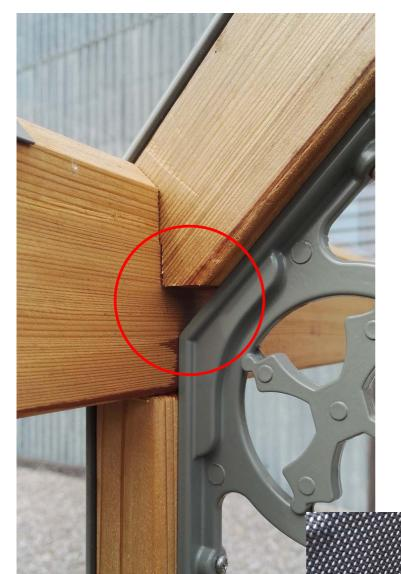
You will find that the universal hooks supplied with the roller blinds will not fit in a satisfactory position at the bottom of the roof bar because of the eaves spandrel. This isn't actually a problem as the ends of the roller blind fit neatly into the hole created behind the spandrel.
