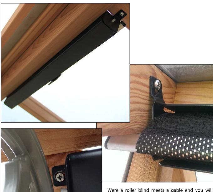
Were a roller blind meets a gable end you will need adjust the direction of the flange. Using an adjustable spanner clamp this onto the flange with the fixing hole in and bend it upwards. You will now be able to fix this inline with the other blinds.
